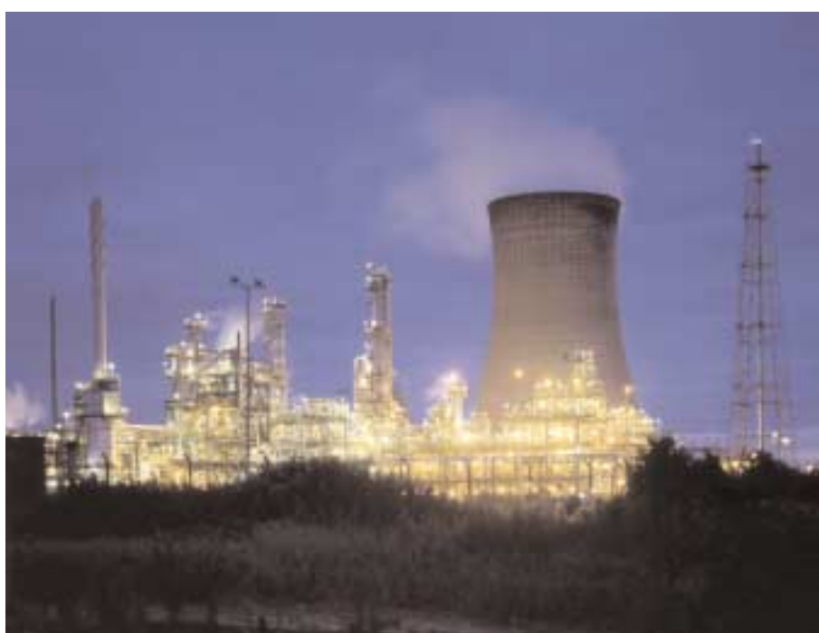
BP Chemicals' plant at Hull, UK has an annual capacity of 250,000 tonnes vinyl acetate monomer
