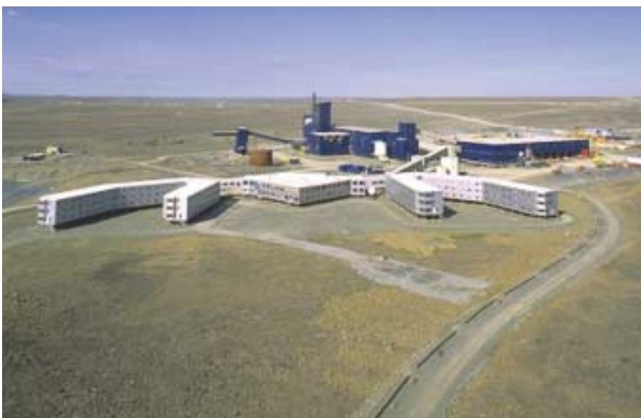
The Falconbridge Raglan mine site in northern Quebec
