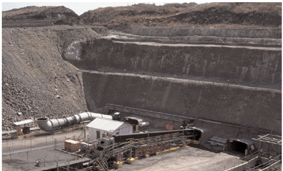
Shallow UG2 ore is mined from this decline shaft at Kroondal Platinum
